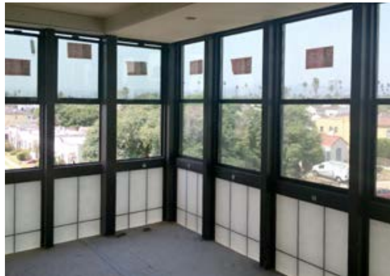
Redondo - Los Angeles, CA, AKA Architects – Los Angeles, CA, Guardian 275® and Glass Mixed Wall Panels
