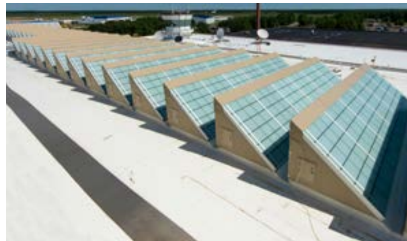
William J. Hughes Technical Center Renovation – Egg Harbor Township, NJ, Guardian 275® Single Slope Skylights
