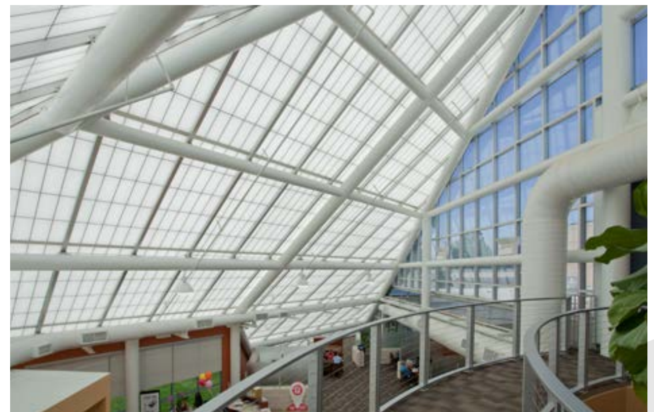
Southwest Airlines Credit Union – Dallas, TX, Guardian 275® Skylight Retrofit
