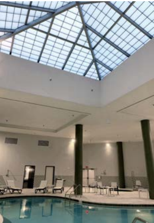
Holiday Inn Express – Panama City, FL, Guardian 275® Pyramid Skylight Replacement
