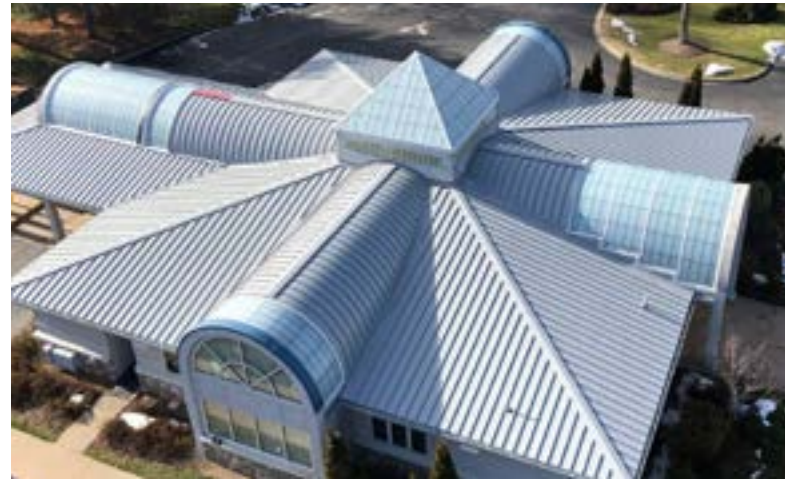
Hometrust Bank – Clyde, NC, Guardian 275® TransCURVE™ and Pyramid Skylight Replacement
