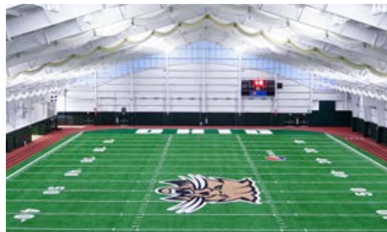
Ohio University - Walter Fieldhouse – Athens, OH., Braun & Steidl Architects, Guardian 275® Wall System, Image by Cory Klein Photography
