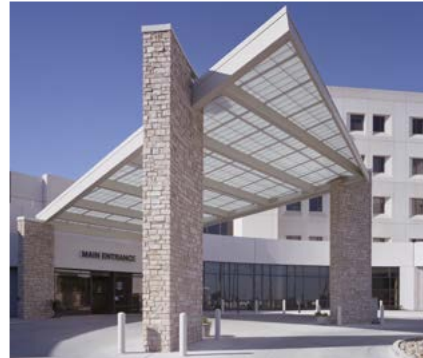
Campbell Memorial Hospital — Gillette, WY, Tractor Glass Company, Guardian 275® Single Slope Canopy
