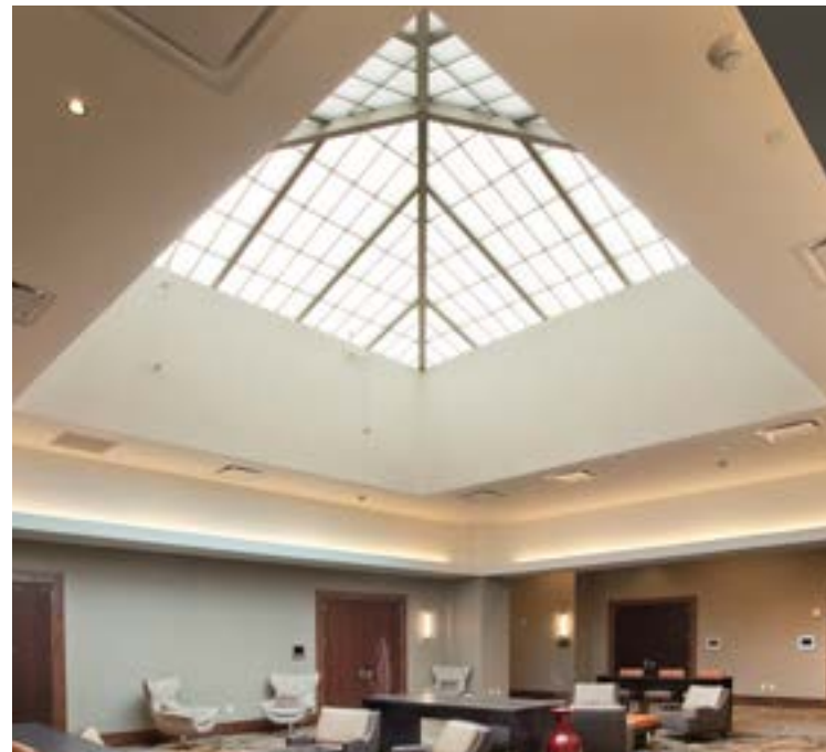
Fitzsimmons Hyatt Hotel – Aurora, CO, TAAG Architects, Guardian 275® Pyramid Skylight
