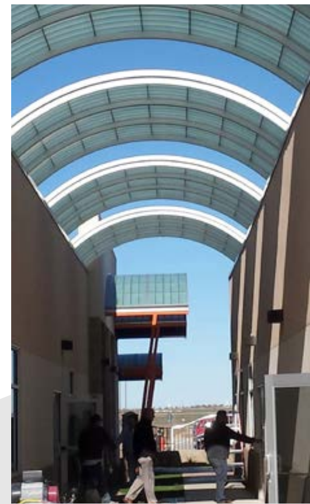
Southwest Cheese – Clovis, NM, NPSR Architects, Guardian 275® TransCURVE™ Canopies
