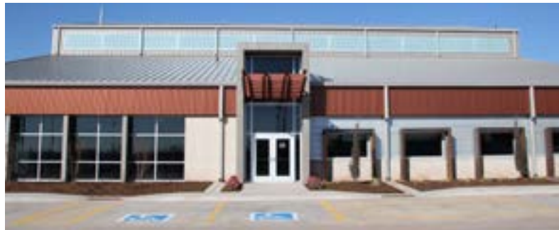
Oklahoma State University - Cooper Engineering Lab – Stillwater, OK, Frankfurt Short Bruza, Guardian 275® Wall System
