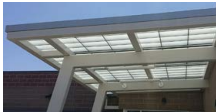
Meridian Public Safety – Meridian, ID, CSHQA, Guardian 275® Single Slope Canopy
