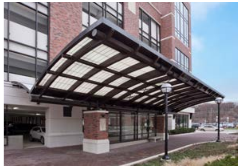
University Parking Garage – Ann Arbor, MI, Walker Parking Consulting, Guardian 275® TransCURVE® Canopy
