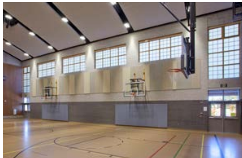
Bend-LaPine Elementary School — Bend, OR, Steele Associates Architects, Guardian 275® Translucent Wall System
