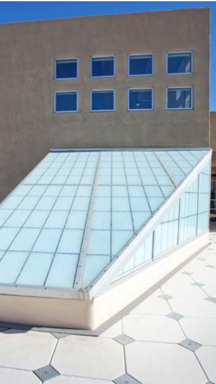
Santa Fe Community College Trades & Advanced Technology Center — Santa Fe, NM, Lloyd & Associates Architects, Guardian 275® Skylight
