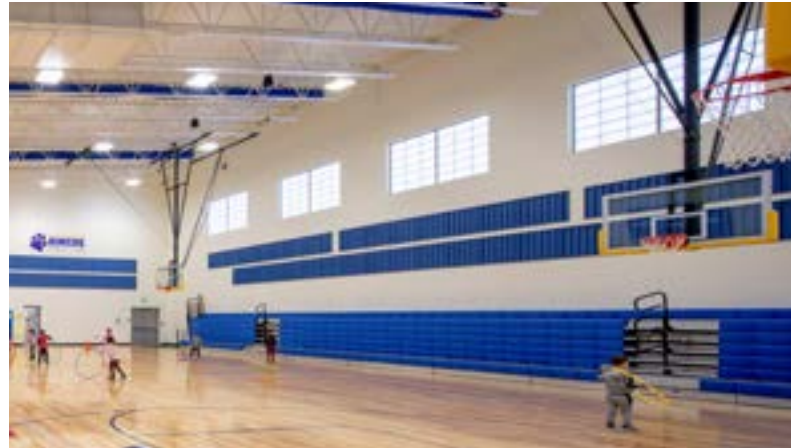
Simcoe Elementary School — Wapato, WA, Architects West, Guardian 275® Wall Systems Image © Firefly Solutions
