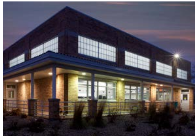
Dept. of Motor Vehicles – Waukesha, WI, Architects Group Ltd, Guardian 275® Wall System
