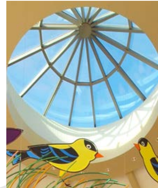
South Dakota Children's Museum — Brookings, SD, Architecture Incorporated, Auburn® Polygon Skylight
