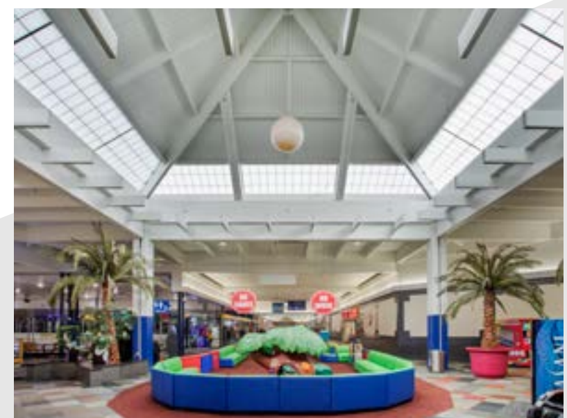
Music City Mall – Odessa, TX, Guardian 275® Skylight Retrofit
