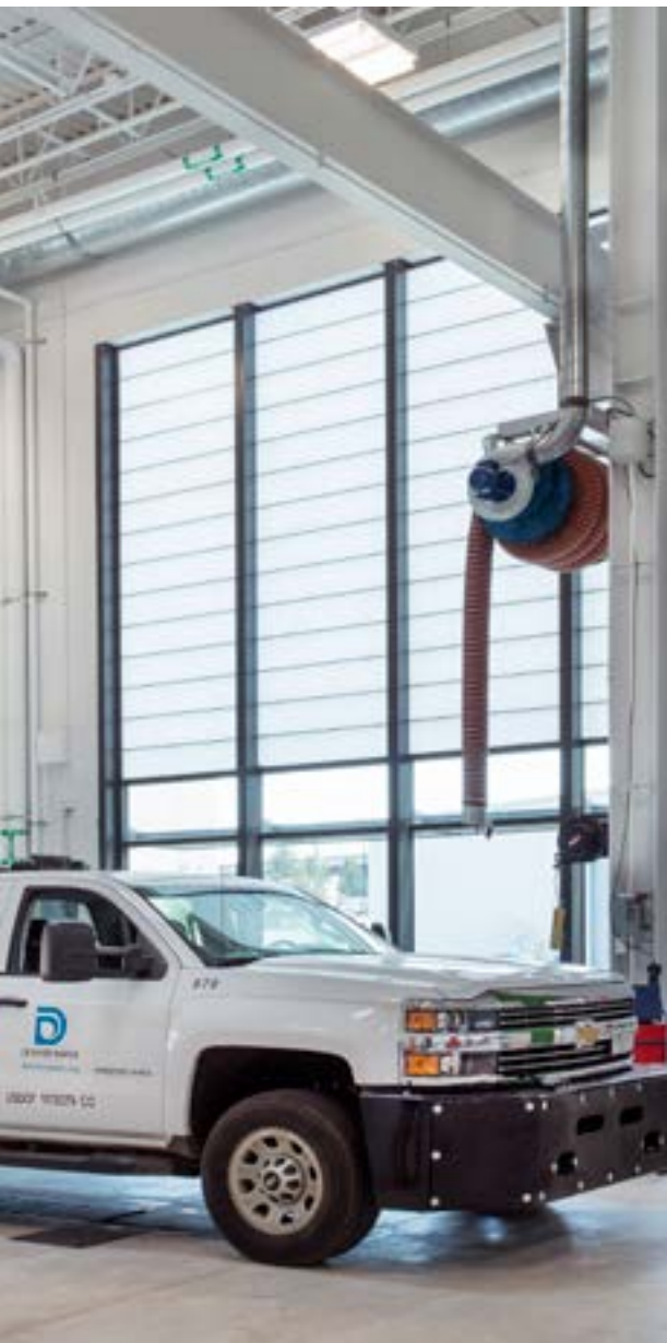
Denver Water Operations Complex – Aurora, CO, RNL – Stantec, Guardian 275® Mixed Glazed Wall System
